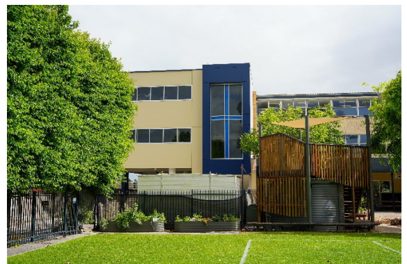
Image - The Stage 1b building nearing completion I refer to above
